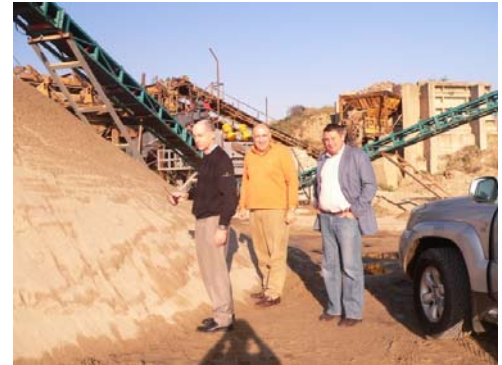
Overseeing the construction progress
