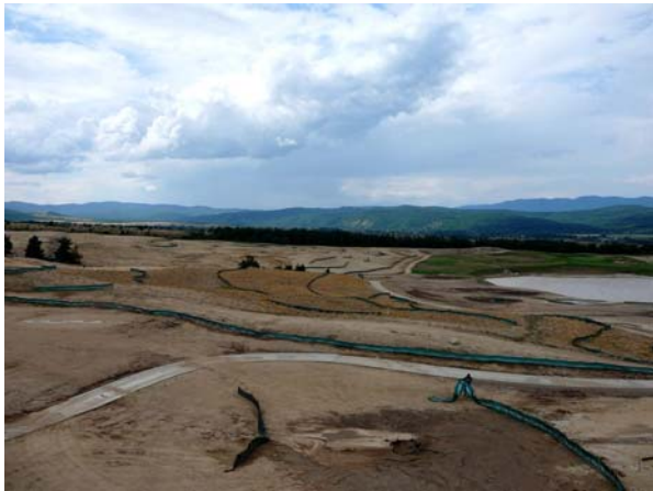
Golf Course under construction
